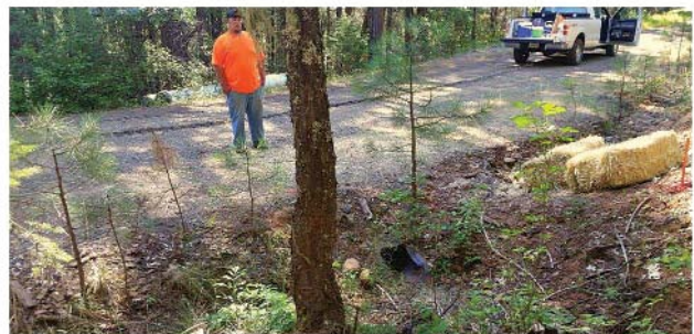
Road 28N66 after 48" corrugated metal pipe was excavated from mainstem of Prospect Creek.
