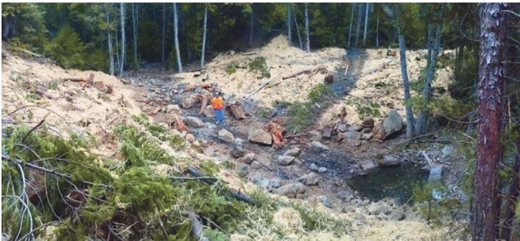
Road 28N66 after 48" corrugated metal pipe was excavated from mainstem of Prospect Creek.
