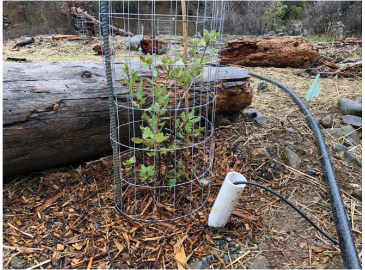
Canyon Live Oak planted at West Weaver Creek Channel and Floodplain Rehabilitation Project.
