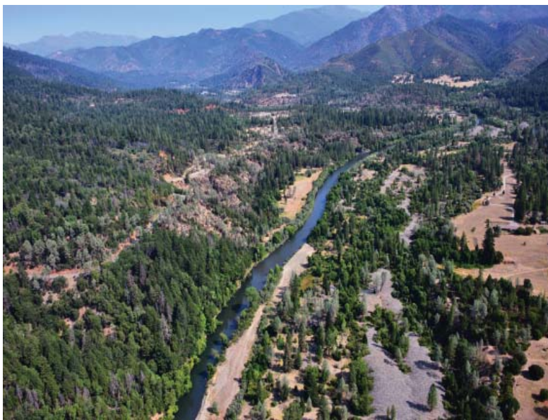
Figure 1. Aerial photography from 2016 of the heavily dredged Deep Gulch and Sheridan Creek project before 2017 construction. The narrow and fast moving channel had limited habitat for rearing young fish successfully.
