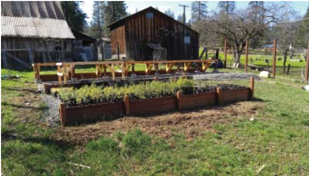
New construction of the Trinity County RCD's native plant nursery.
