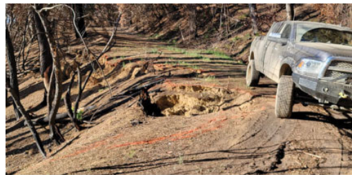
A replaced culvert allowing for improved water flow without causing road erosion
