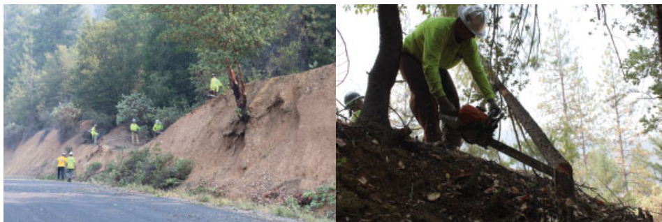
Crews construct a roadside shaded fuel break along Steiner Flat Road.
