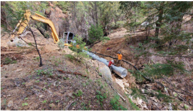
Installation of a culvert at an eroded stream crossing
