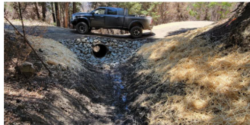
A replaced culvert allowing for improved water flow without causing road erosion
