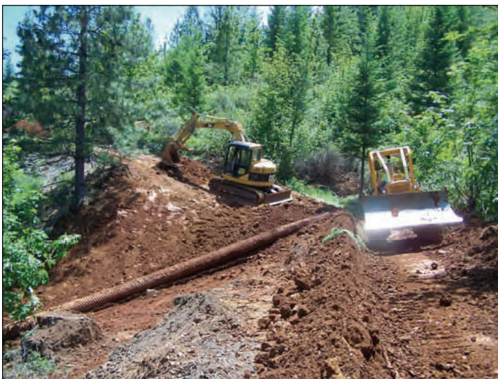
Browns Road Decommission
