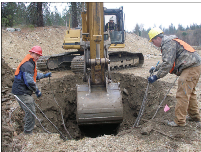
TCRCD crew assisting excavator
