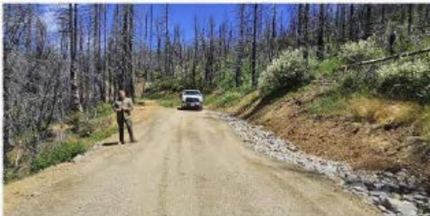
Perforated pipe drains, then rip rap installed in ditch and across road to improve drainage at spring
