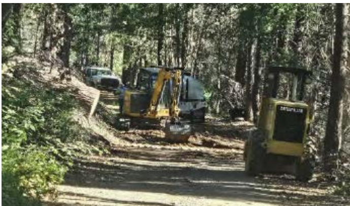
Perforated pipe drains, then rip rap installed in ditch and across road to improve drainage at spring
