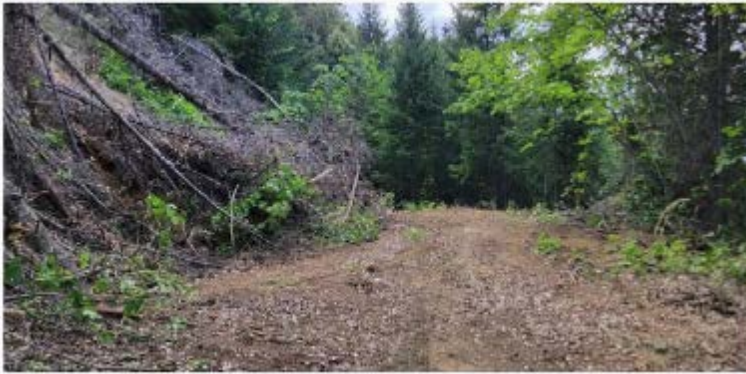
Before and after clearing 5N04 road
