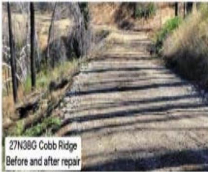
2512 NWI 0.50 Fill failure repair September 2024
