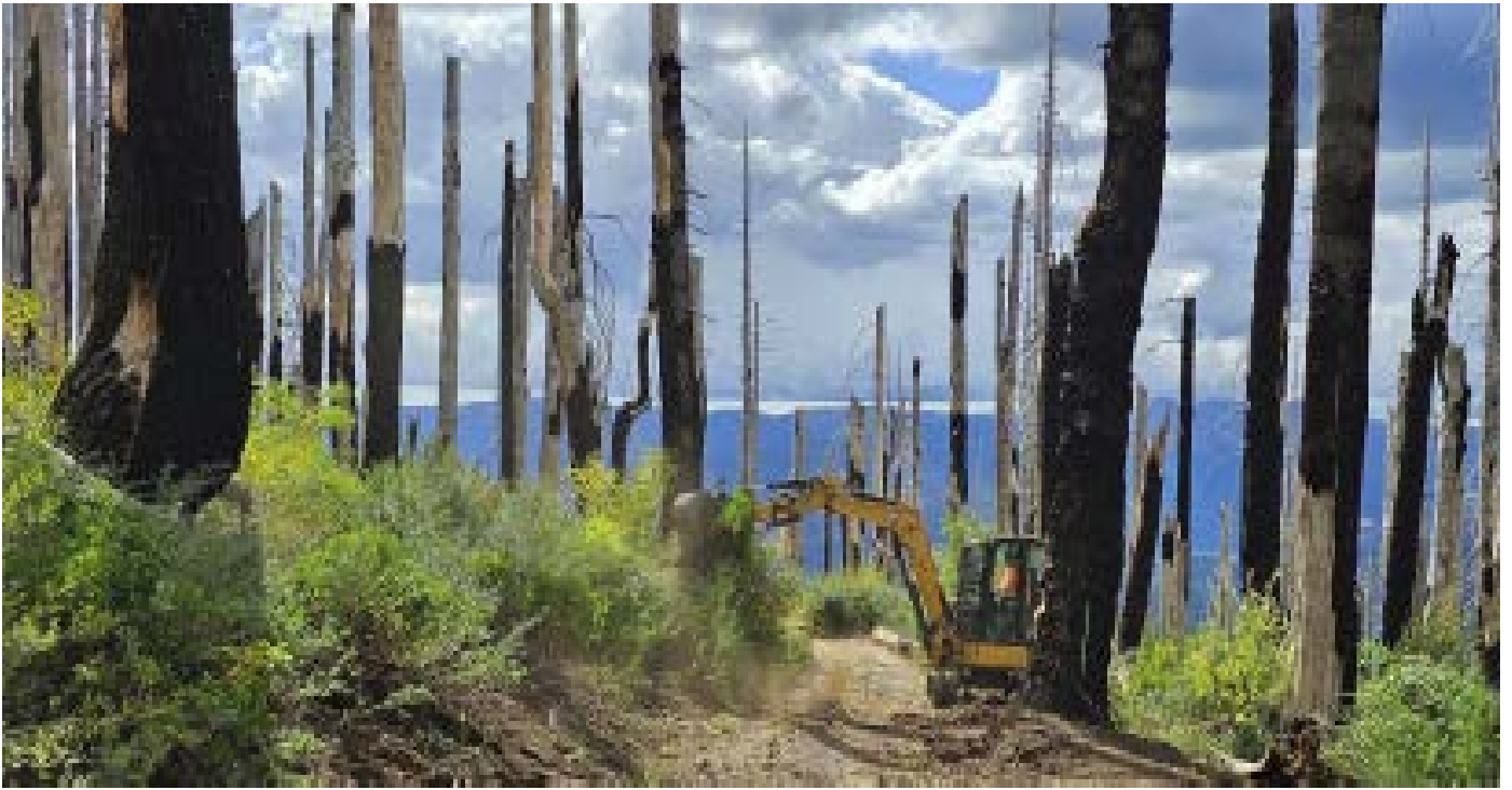
Clearing logs and brush from road on north side of 1S05 Pickett Peak
