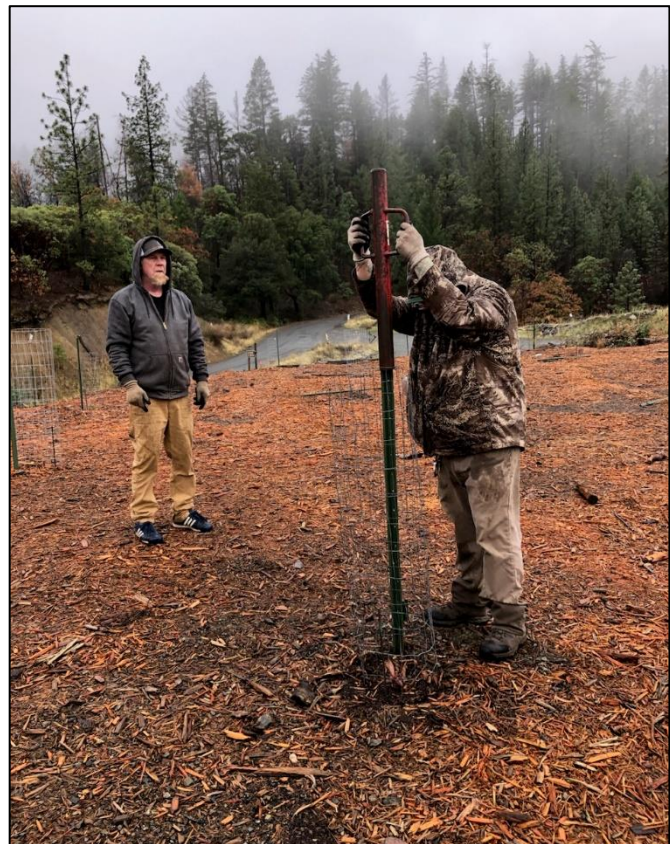
Tom Asgeirsson and Tom Robertson reinforcing plant cages at the Big French Creek Disposal revegetation site.
